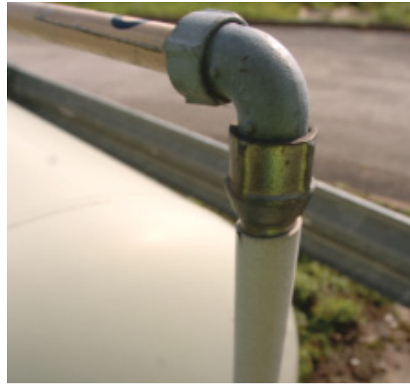
Pipework protected from last collar before entering ground
